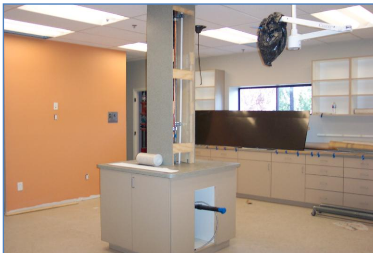
TREATMENT AREA PROGRESSING: Almost Ready to Open!
