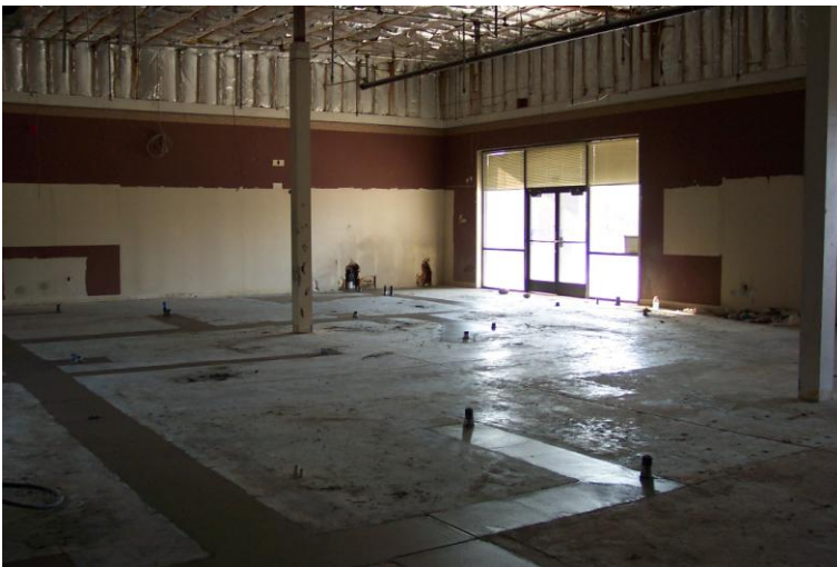
BEFORE THE WALLS: Plumbing Installation in Early July
